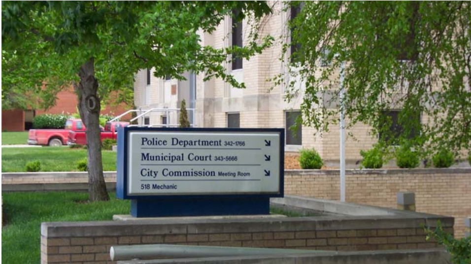
Entrance to Municipal Court from outside the Civic Auditorium, looking north.
